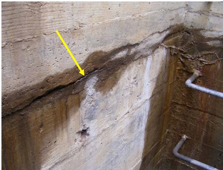
Dam Inspection Manhole: Photo 42
