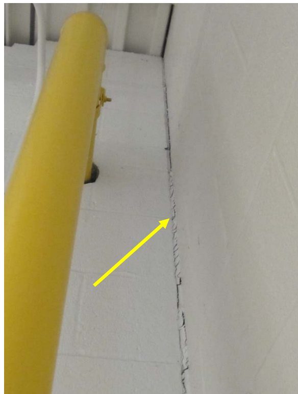
Building 19 2005 Addition: Photo 22
