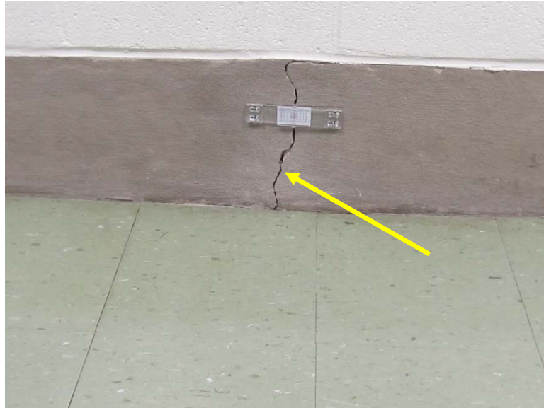
Building 19 2005 Addition: Photo 19
