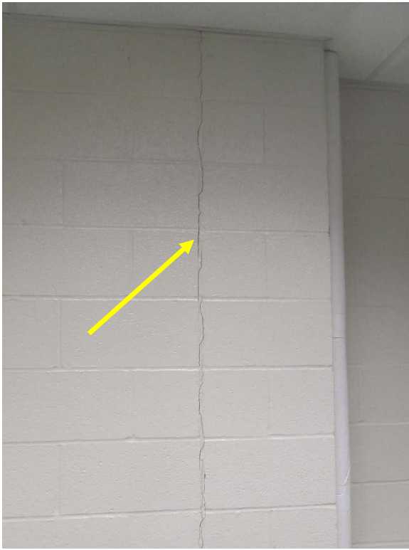
Building 19 2005 Addition: Photo 21
