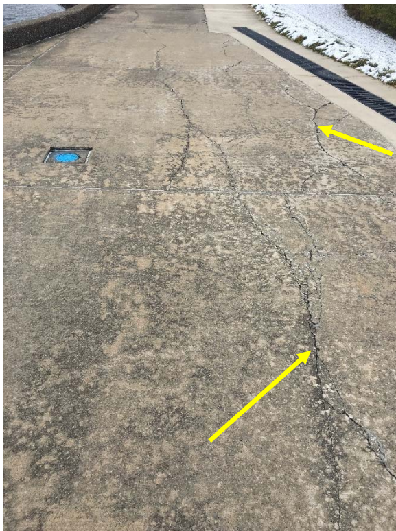
Dam Roadway Slab: Photo 39
