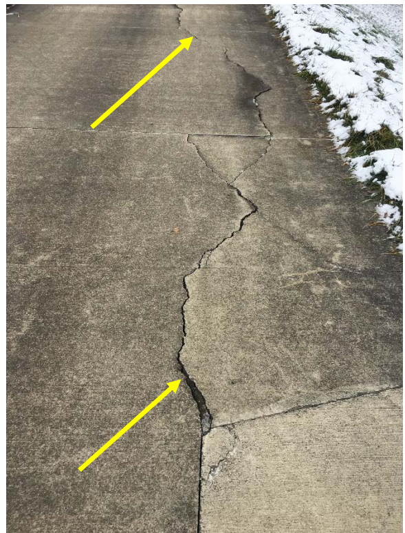
Dam Roadway Slab: Photo 40
