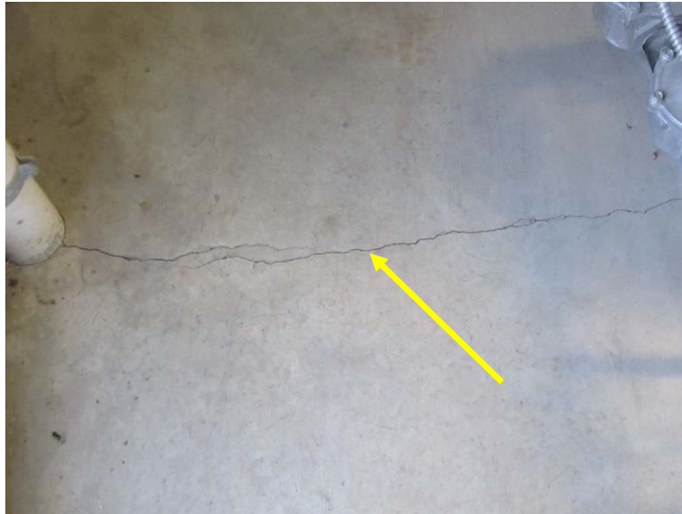
Building 19 2005 Addition: Photo 24
