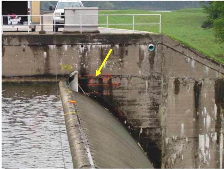
Dam Spillway West Training Wall: Photo 41
