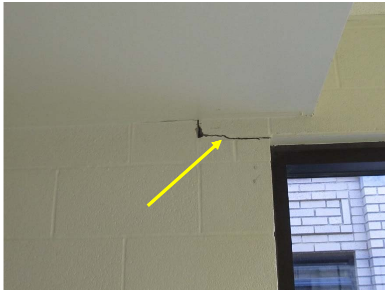
Building 19 2005 Addition: Photo 18
