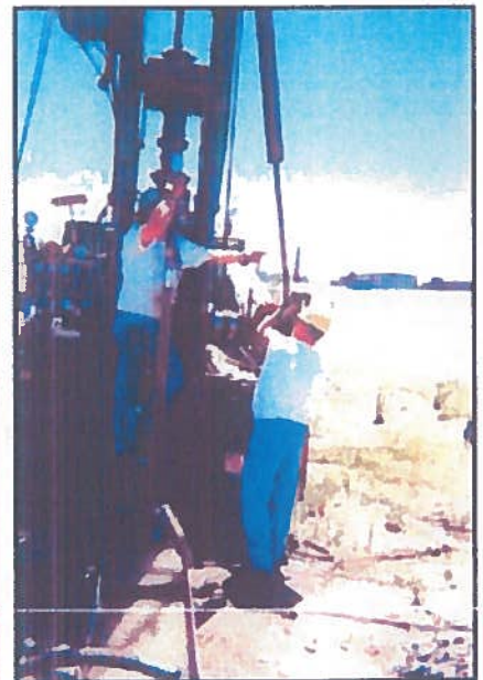
Attaching SPT to Instrumented Rod Section
