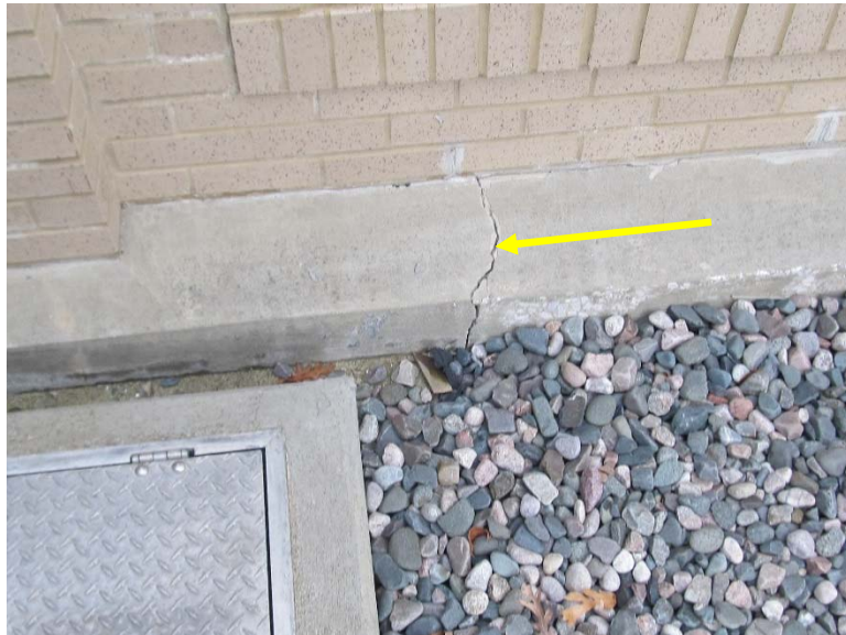
Building 19 2005 Addition: Photo 20
