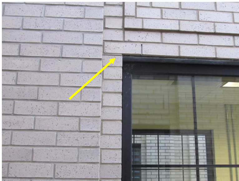
Building 19 2005 Addition: Photo 25
