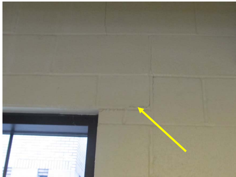
Building 19 2005 Addition: Photo 23
