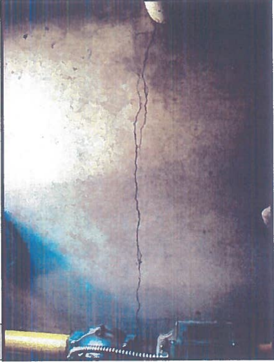
Floor Slab Cracking
